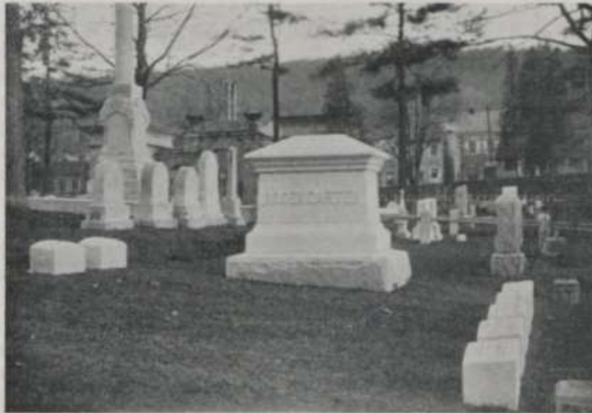
The sizes of this Barclay Monument are: Cap, 4-8x2-10x1-4; Die, 4-9x2-2x1-10; Base, 4-8x2-10x1-0; B. Base, 5-7x3-9x1-4.
