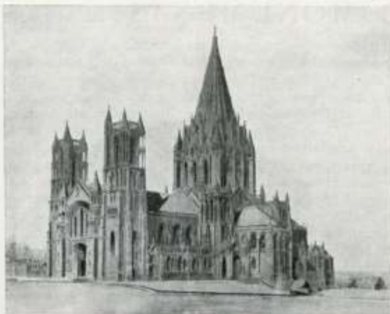
DESIGN FOR CATHEDRAL OF ST. JOHN THE DIVINE. Heins & La Farge, Architects.
