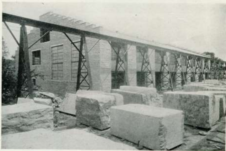
Exterior of new mill of F. W. Steadley & Co., Inc., constructed of Colonial Grey Veined and Veinless Marble with steel roof, window frames and equipped throughout with concrete floors, making it absolutely fireproof.
