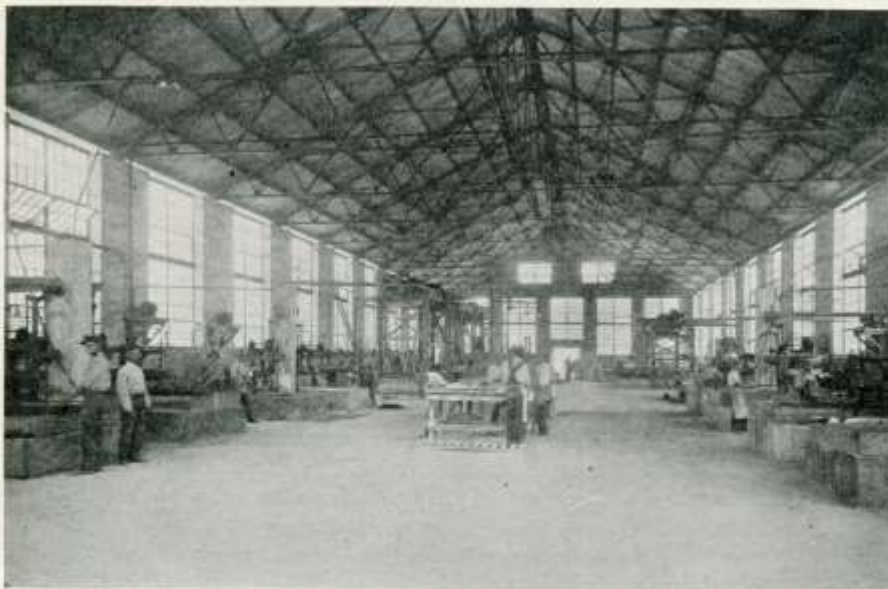
Interior of new marble finishing plant of F. W. Steadley & Co., Inc., devoted exclusively to finishing marble for interior work.
