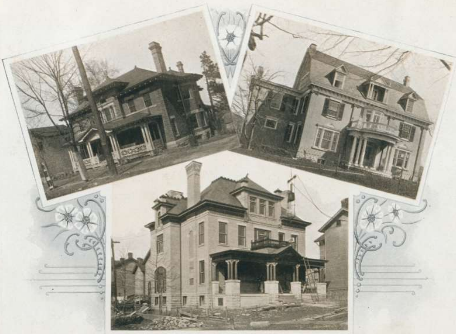
Residences Recently Erected in Different Parts of the United States Covered with Genuine Bangor Excelsior Slate.
