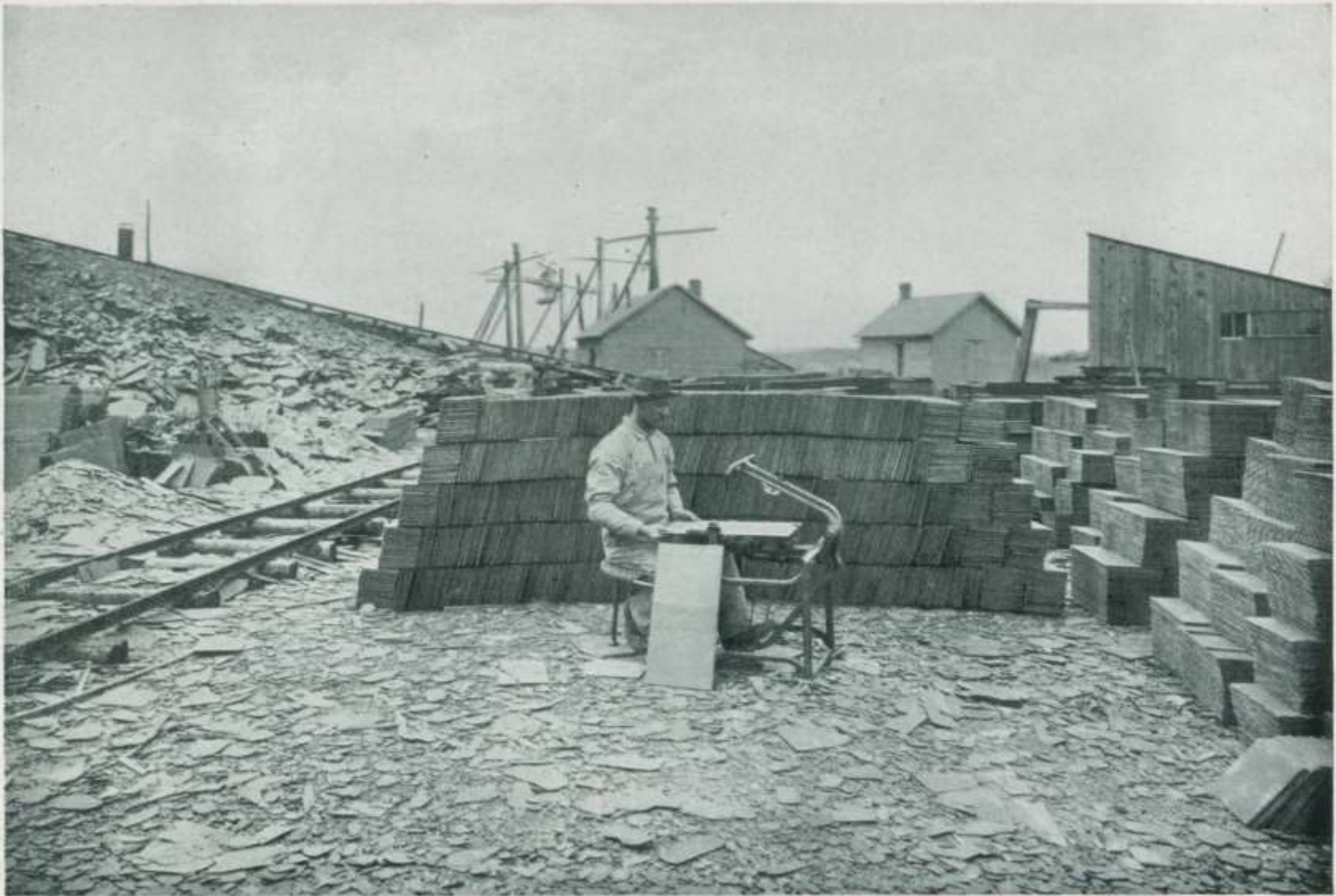
Workman Punching Slate, Ready to Lay.
