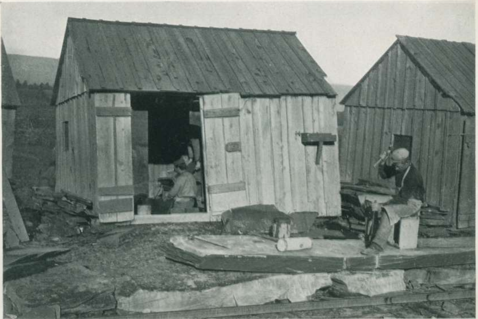
Workmen Sculpting and Splitting Blocks of Slate.
