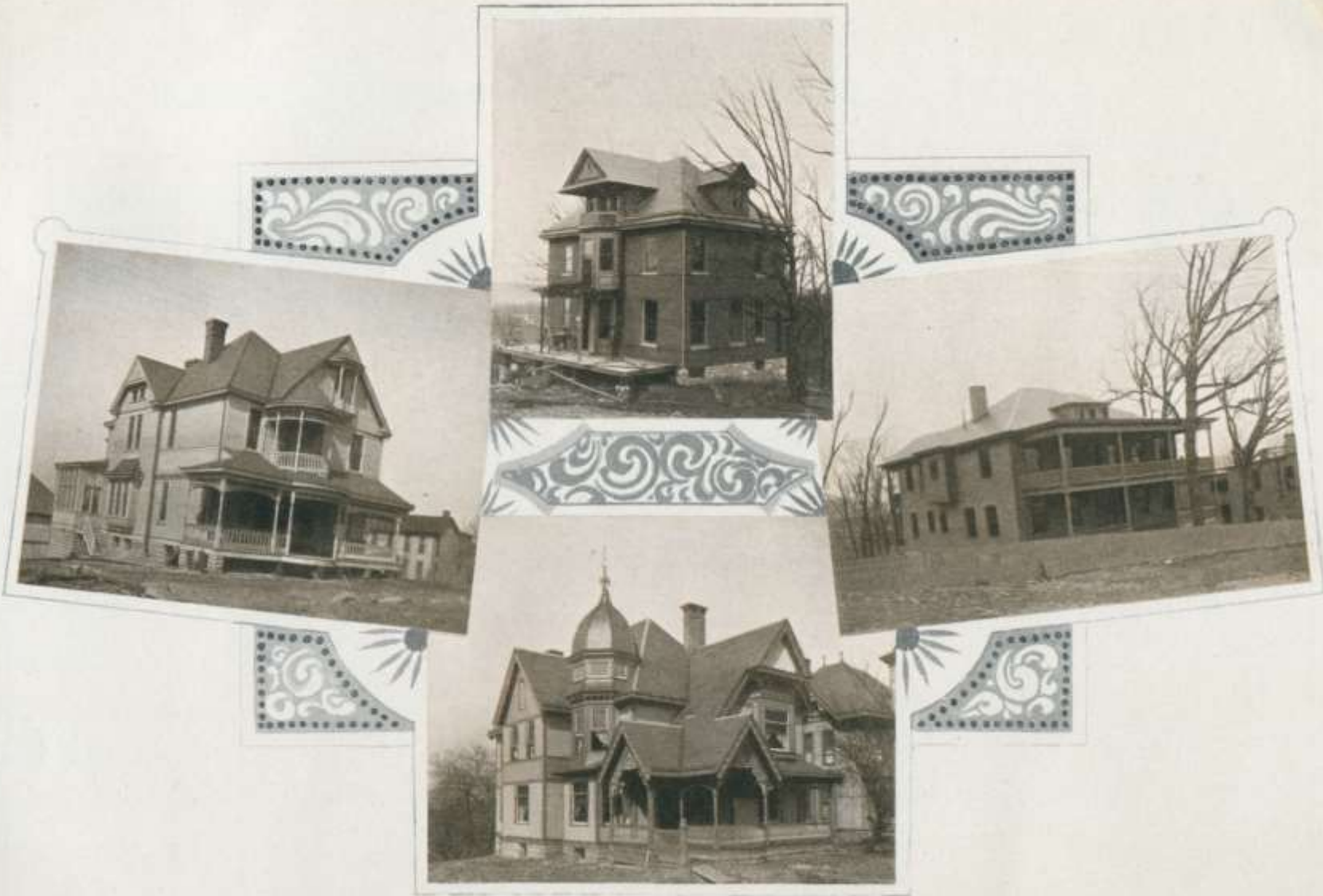
Residences Recently Erected in Different Parts of the United States Covered with Genuine Bangor Excelsior Slate.
