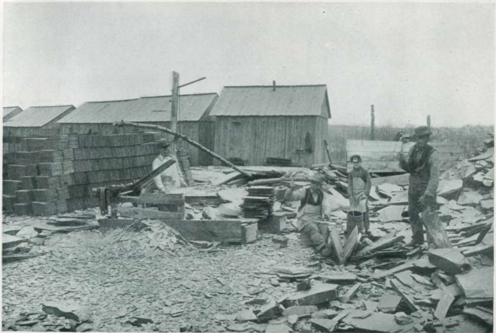
Workmen Splitting and Dressing Slate to Size.
