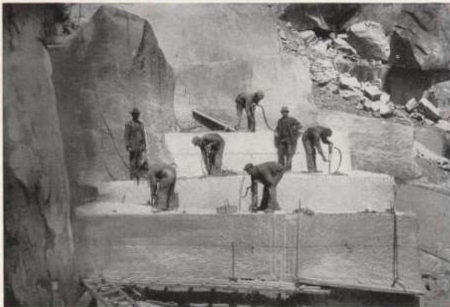
Sullivan "D-15" Hammer Drills in the Bay View Quarries.
