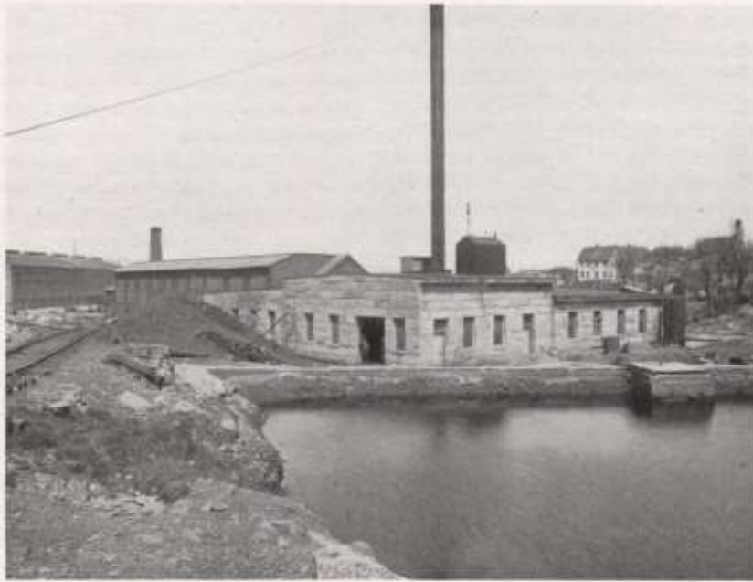
Bay View powerhouse and finishing plant of the Rockport Granite Co.
