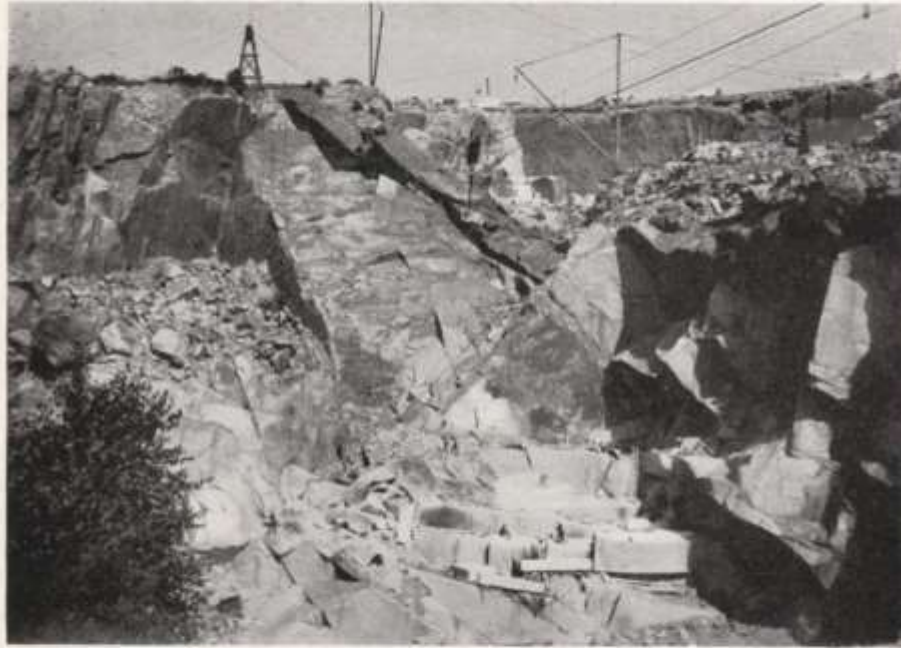
A general view of one of the quarries.
