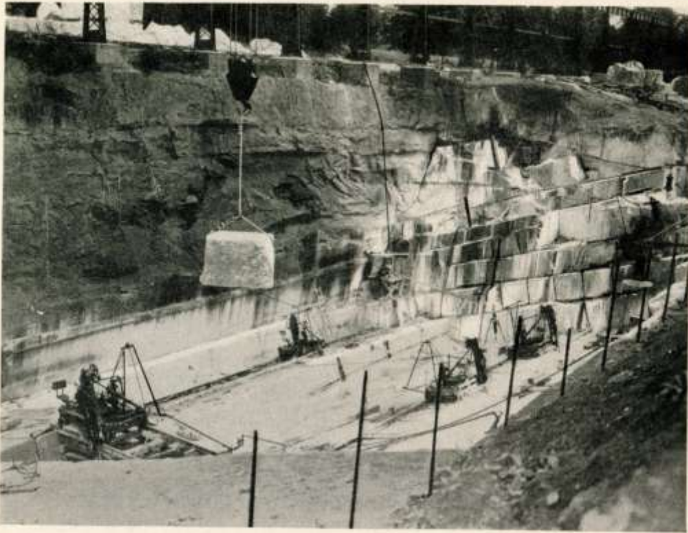
The Main Quarry Pit, Missisquoi Marble Co.
