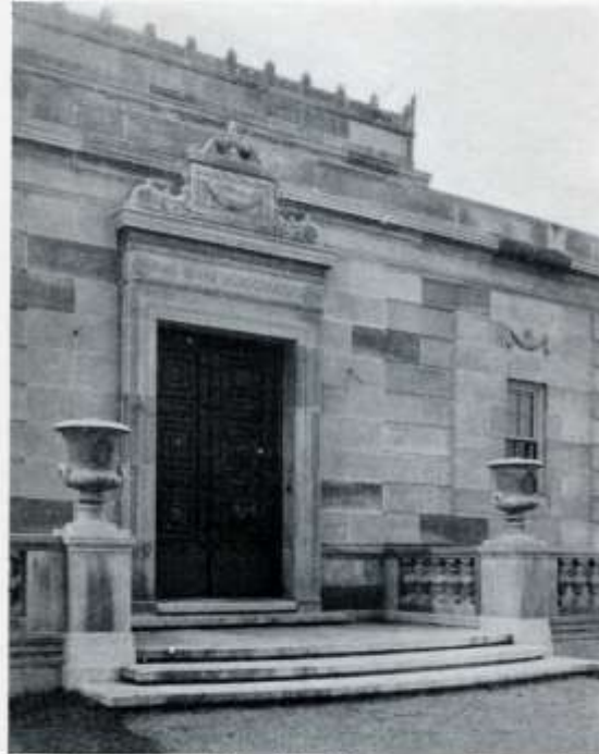
Main Entrance of new Fire Alarm Headquarters, Boston, showing the carved work, urns and decorative details in the same material as the walls. O'Connell & Shaw, architects.
