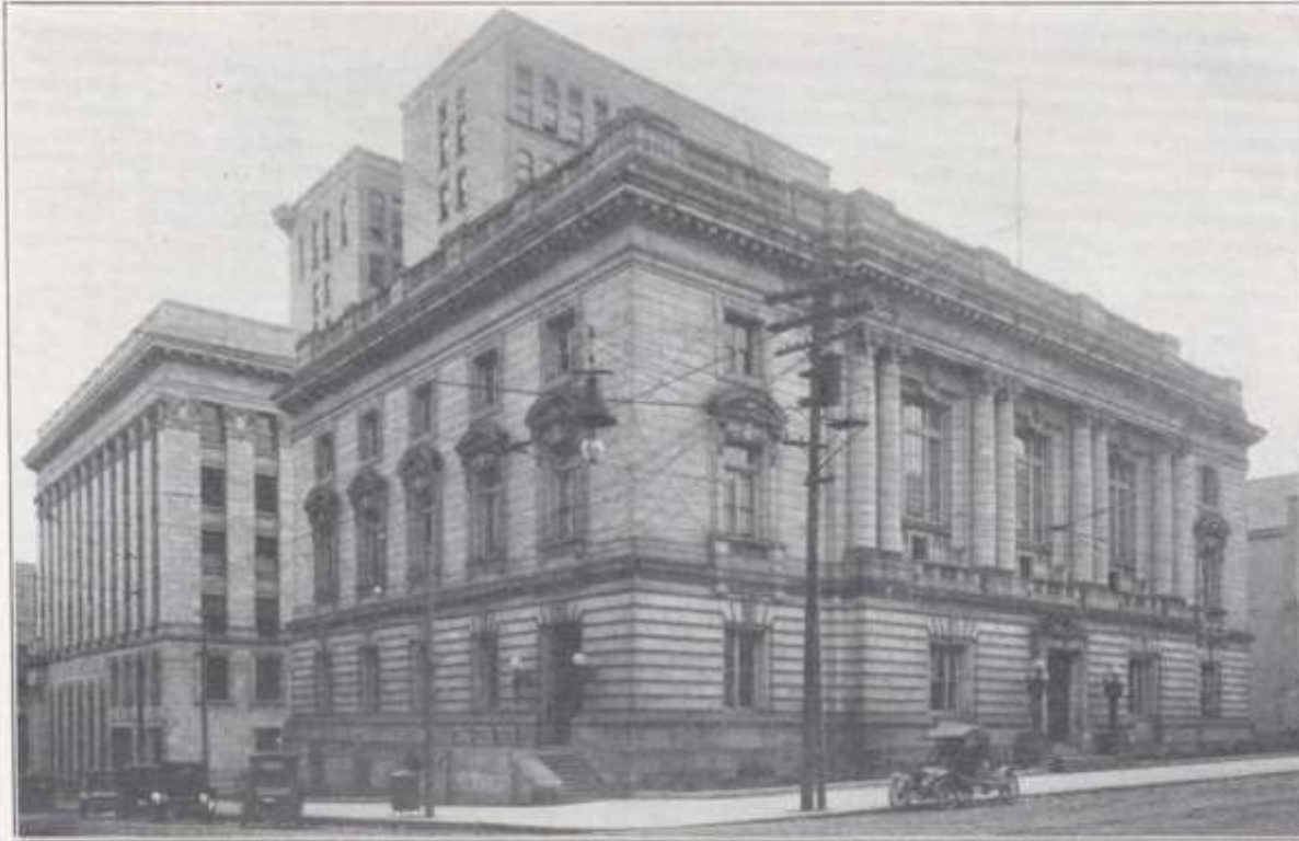
UNITED STATES POSTOFFICE, Wheeling, W. Va. Superstructure of Stone Mountain Granite. 34,000 cubic feet. Marsh & Peter, Architects
