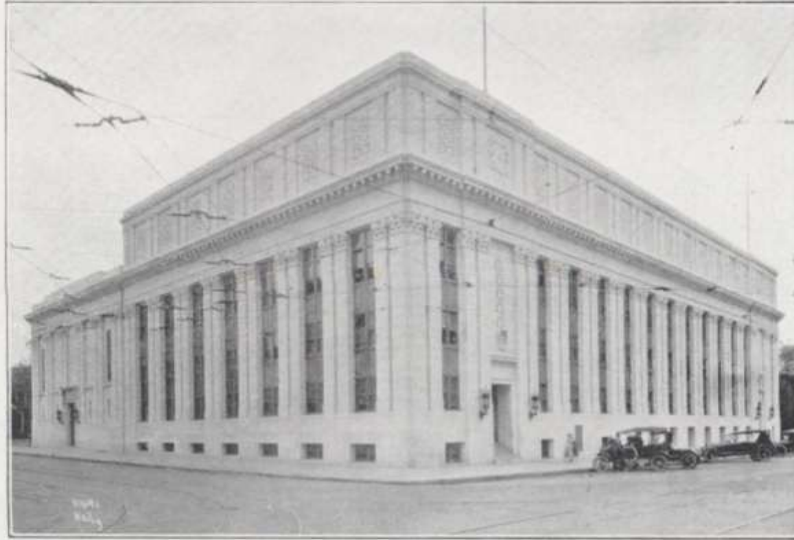
MASONIC TEMPLE, Birmingham, Ala. Warren & Knight, H. B. Wheelock, Architects
