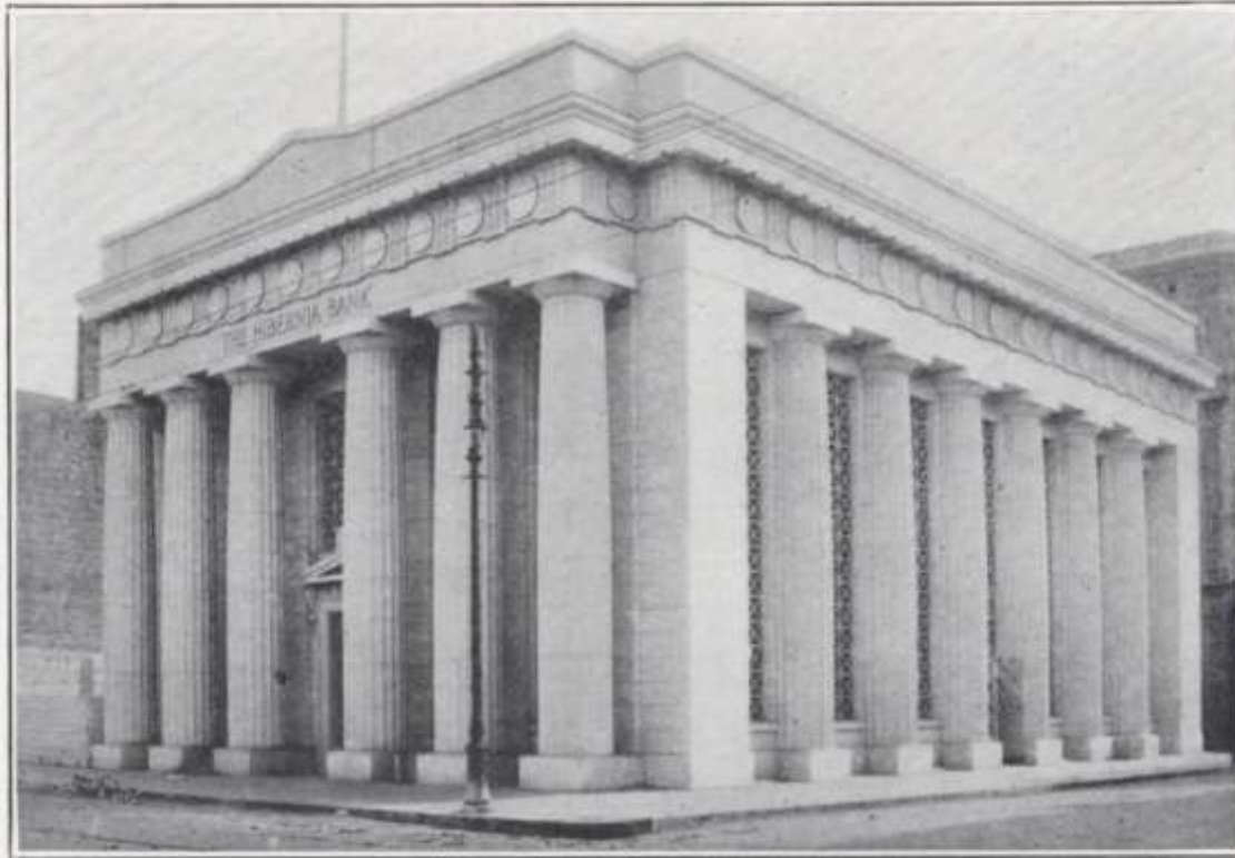
HIBERNIA BANK BUILDING, SAVANNAH, GA. Stone Mountain Granite. 12,500 cubic feet of cut granite Mowbray & Uffinger, Architects
