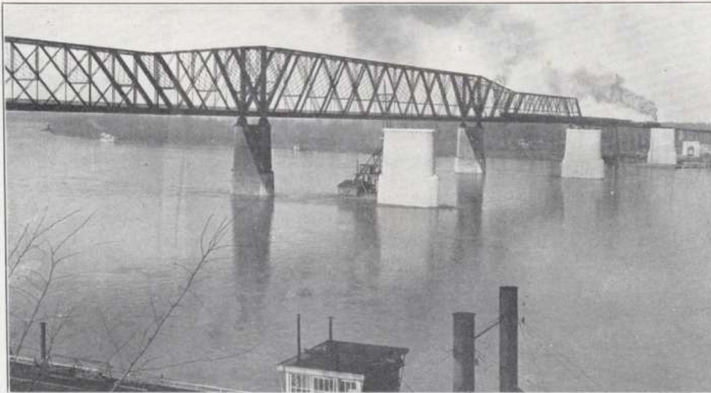
Piers of Stone Mountain Granite of the new Harahan Bridge over the Mississippi River at Memphis, Tenn. Union Bridge & Construction Co., General Contractors. Ralph Modjeski, Engineer, Chicago. Contains 255,600 cubic feet of cut granite.
