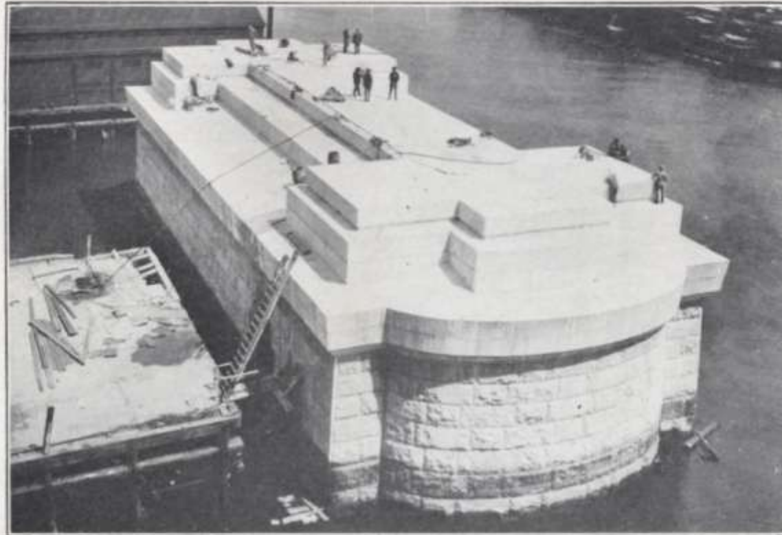
ONE OF THE TWO MAIN PIERS OF THE DELAWARE RIVER BRIDGE BETWEEN PHILADELPHIA, PA., AND CAMDEN, N. J. Containing 171,000 Cubic Feet Cut Stone Mountain Granite.
