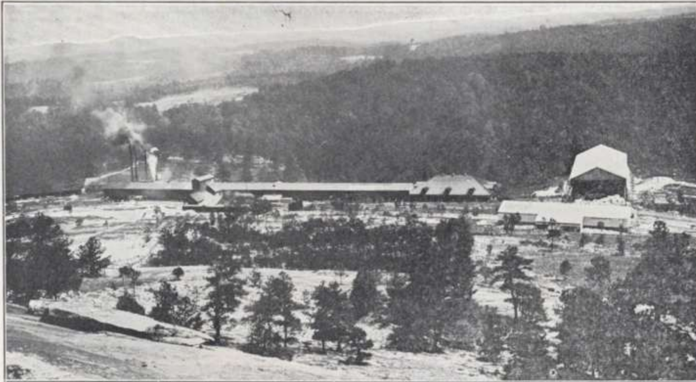
View taken from a point 150 feet up the Mountain slope, showing the Power Plant, Cutting Sheds, Blacksmith Shops and Crushing Plant. Since this picture was taken, Steam Power was abolished and replaced by Electric Power furnished by the Georgia Railway & Power Co., and brought from Tallulah Falls, Ga.
