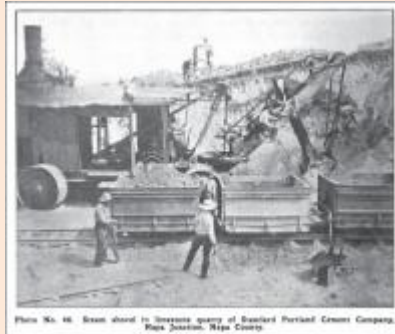
Steam shovel in limestone quarry of Standard Portland Cement Company (circa 1916)
