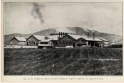
Works of the Standard Portland Cement Company at Napa Junction. (Ill. No. 79, circa 1906)
