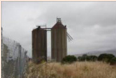
These silos were added by the Basalt Rock Co. in the late 1940s to early 1950s after the cement plant shut down, according to Linda Luippold.
