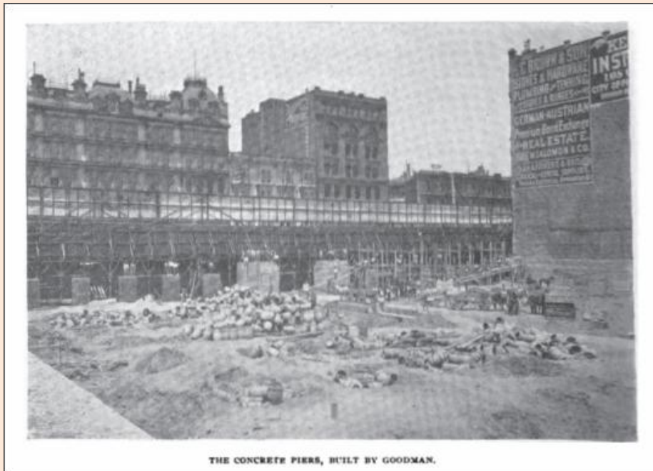
THE CONCRETE PIERS, BUILT BY GOODMAN.
